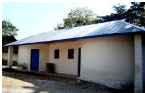
Completed trainee hostel
